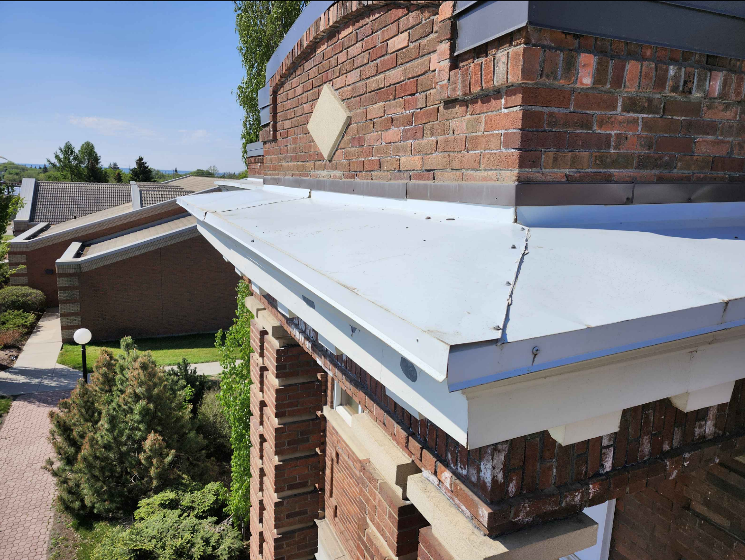
PROVISIONAL WORK 3: CORRECTION OF SAG AT MAIN ENTRANCE CORNICE
