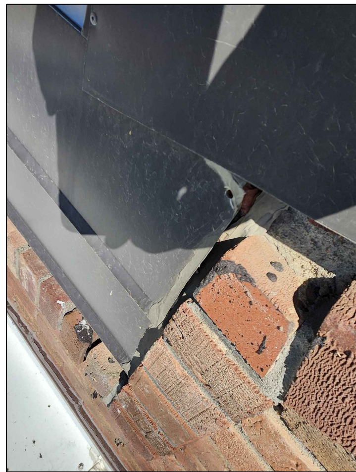
GAP AT VERTICAL PARAPET FLASHING
