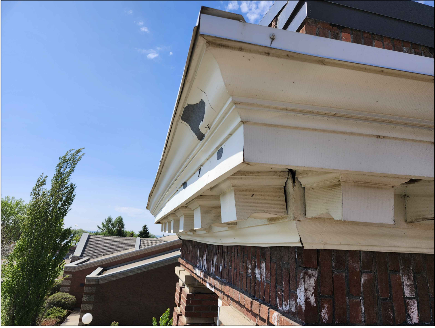
PROVISIONAL WORK 3: CORRECTION OF SAG AT MAIN ENTRANCE CORNICE
