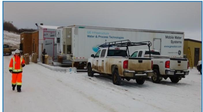
The GE pre-filtration system allow approximately 40 litres per second of water to be processed and filtered at the F.E. Holliday water treatment plant. Additional testing was
