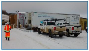
treatment plant. The GE pre-filtration system allow approximately 40 litres per second of water to be processed and filtered at the F.E. Holliday water treatment plant. Additional testing was
