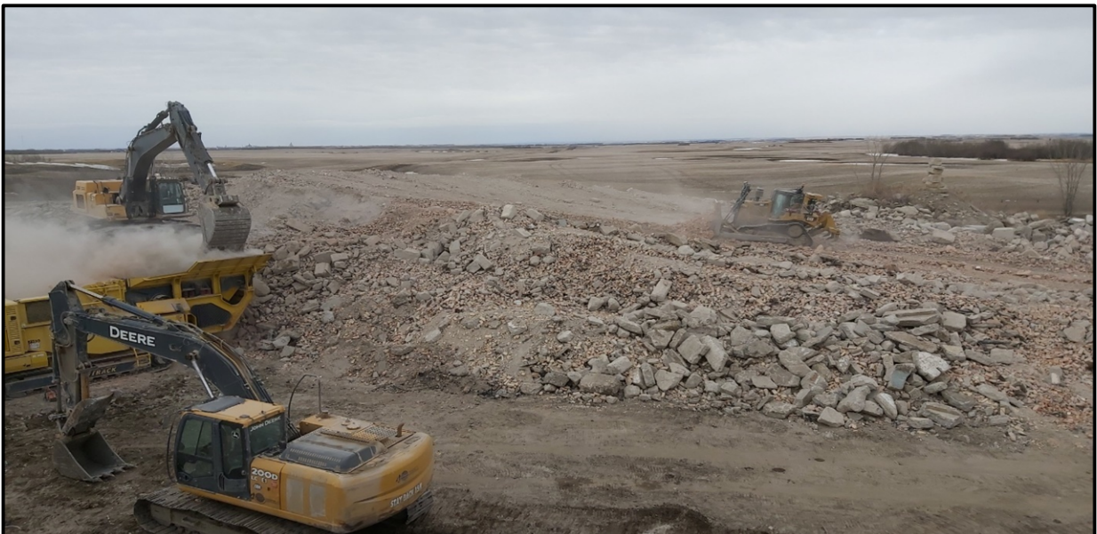
Photo 2. Crushing of Concrete pile in 2021
