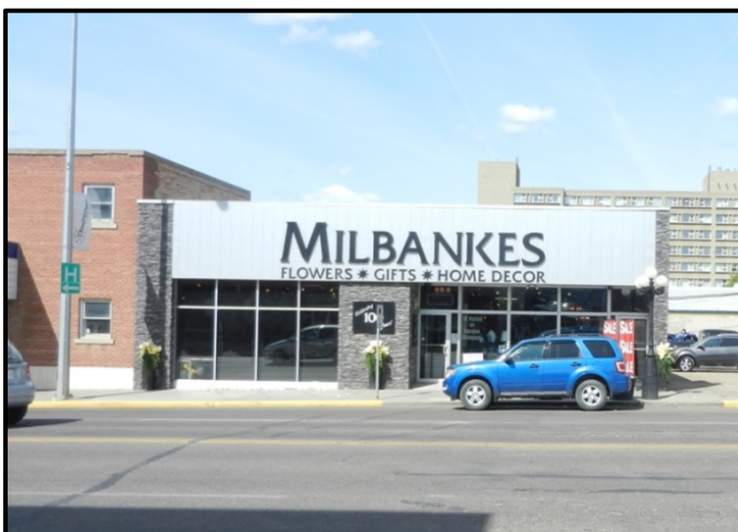
Figure15: Existing Well Maintained Building
