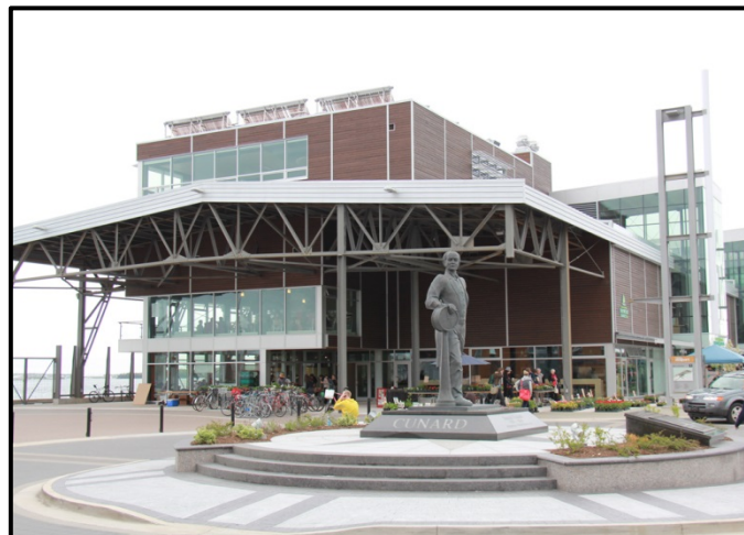
Figure 52: Halifax Seaport Farmers Market (RCS Construction)
