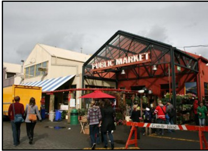
Figure 48: Metal and Glass Cladding Materials (Inside Vancouver)
