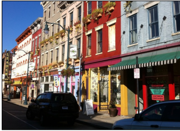
Figure 30: Colourful Street Façades (jathanandheather.com)
